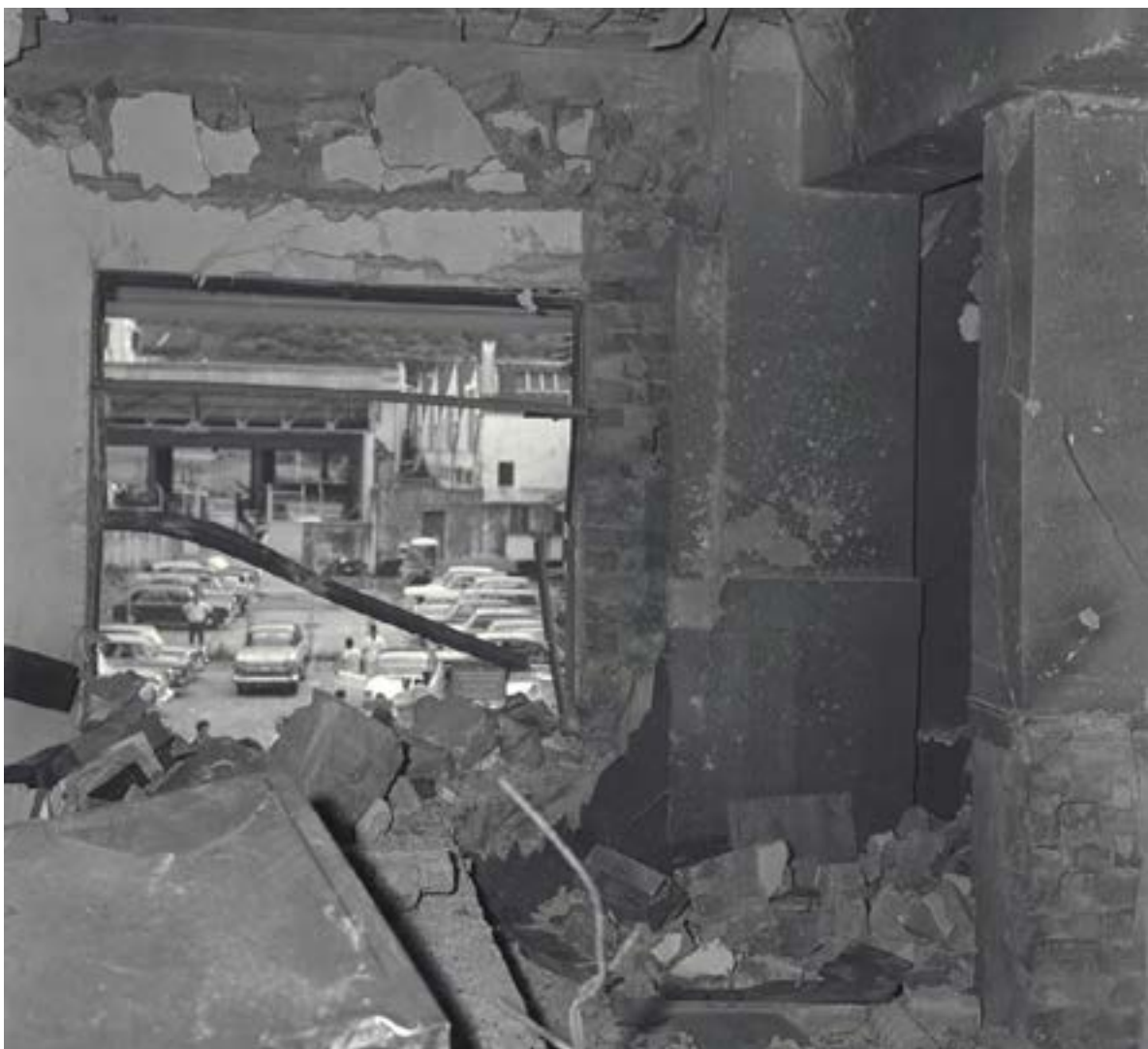
The concrete wall separating the stairway and the correspondence room of the Hong Kong and Shanghai Bank was completely destroyed by the bomb, exposing a side of the bank's car park.
